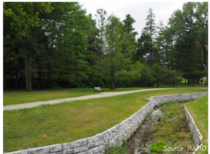
Figure 8.34 Limestone wall stream bank stabilization in Read Park
