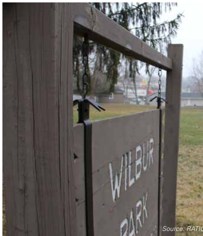
Figure 8.10 Detail of identification sign. The sign is attached to the wood frame with wrought iron brackets and a black chain.
